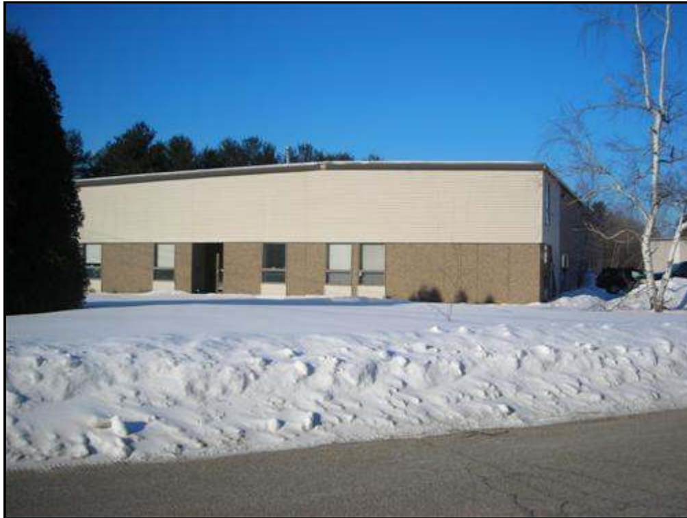
Front view of building.
