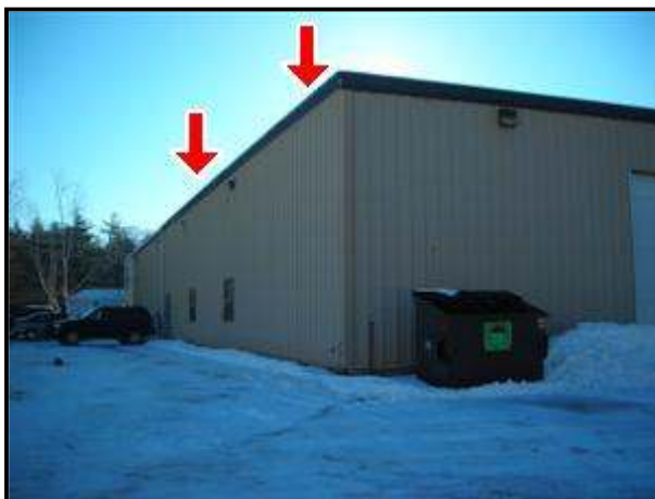
1.2 Picture 1 Install gutters and downspouts.
