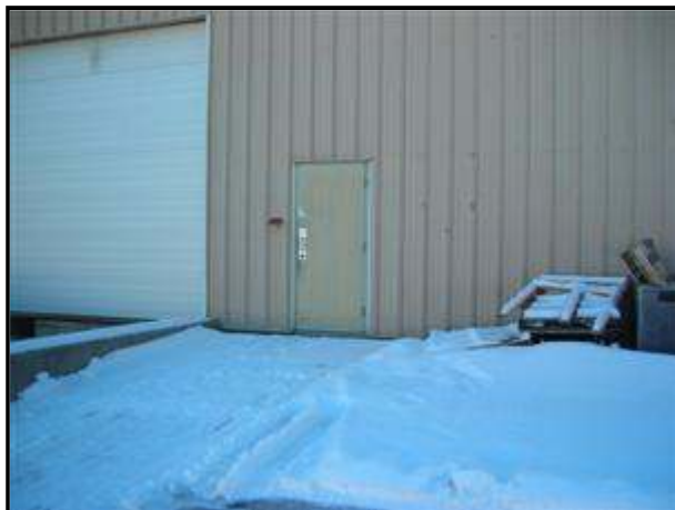
2.1 Picture 3 Upgrade door.
